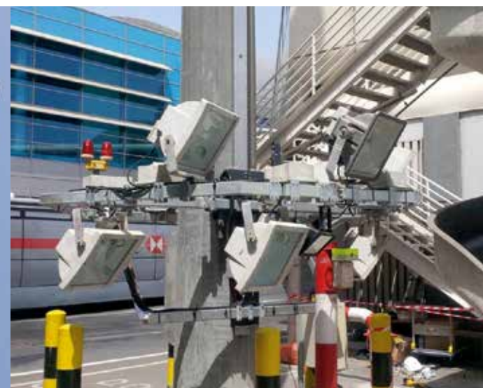
Dubai Airport: Retrofitting of existing high mast with NivaLift-L-750
