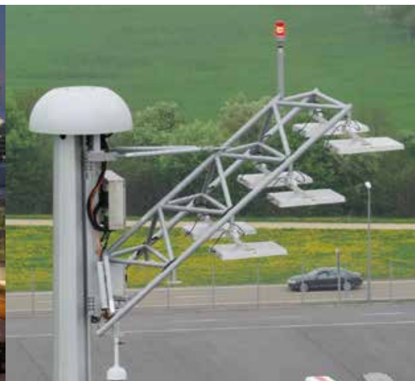
Munich Airport, Germany / Conventional and new LED floodlights
